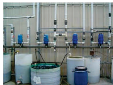
Tanks of fertigation system containing nutrient solutions
